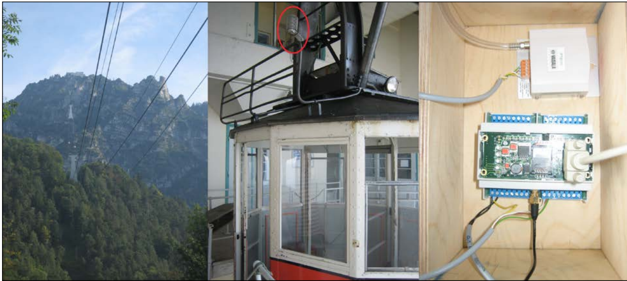
Fig. 10 Cable car route (left), cable car cabin with sensor screen (centre) and GSM data logger with pressure sensor (right)
