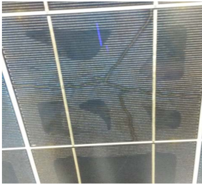
Fig. 4: Particular of one of the cells of the module shown in Fig. 3, highlighting the presence of decorated micro-cracks with burnmarks and discoloration of finger grids, in combination with a possible delamination of the encapsulant.
