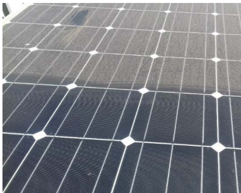
Fig. 5: Soiling can account up to 60% current and power losses.
