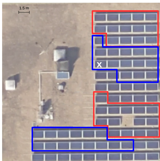
Figure 5.5 – PV installation at the EPFL laboratory (GPS coordinates 46.52-N, 6.56-E). The strings indicated with blue color are connected to C1 and the strings indicated with red color are connected to C2. The white cross indicates the panel where the temperature sensor and the pyranometer are installed.
