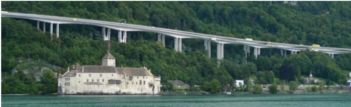
Figure 6. Chillon Viaducts along Lake Geneva.
