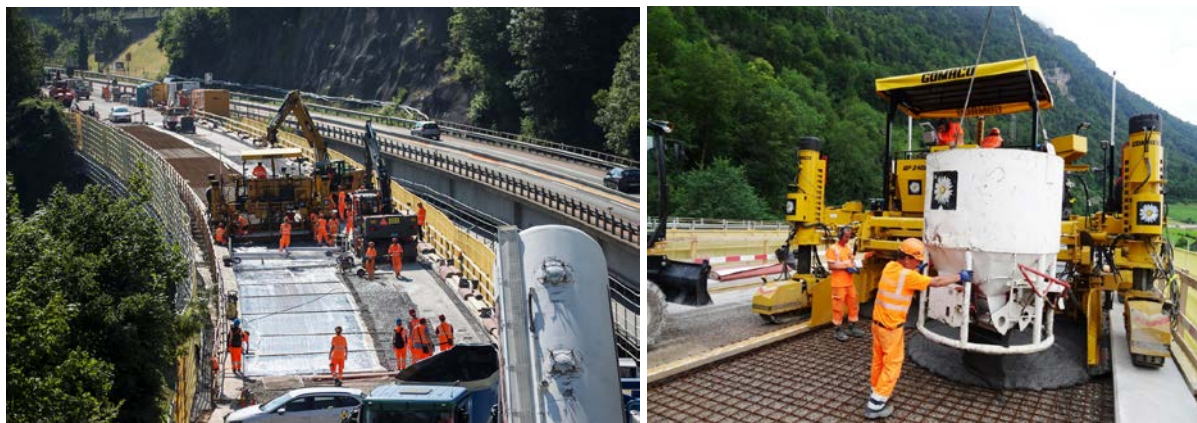
Figure 10. General view of construction site on 12 th of July 2018 (left; Photo A.Wey keystone), and UHPFRC casting using a finisher (right).
