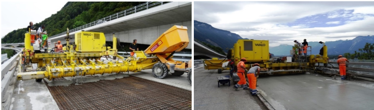
Figure 8. UHPFRC casting finisher (left) and fresh UHPFRC layer after casting (right).
