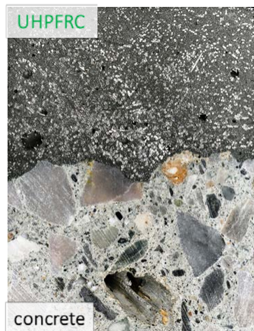
Fig. 1. UHPFRC – concrete core showing the obvious difference between the two materials.
