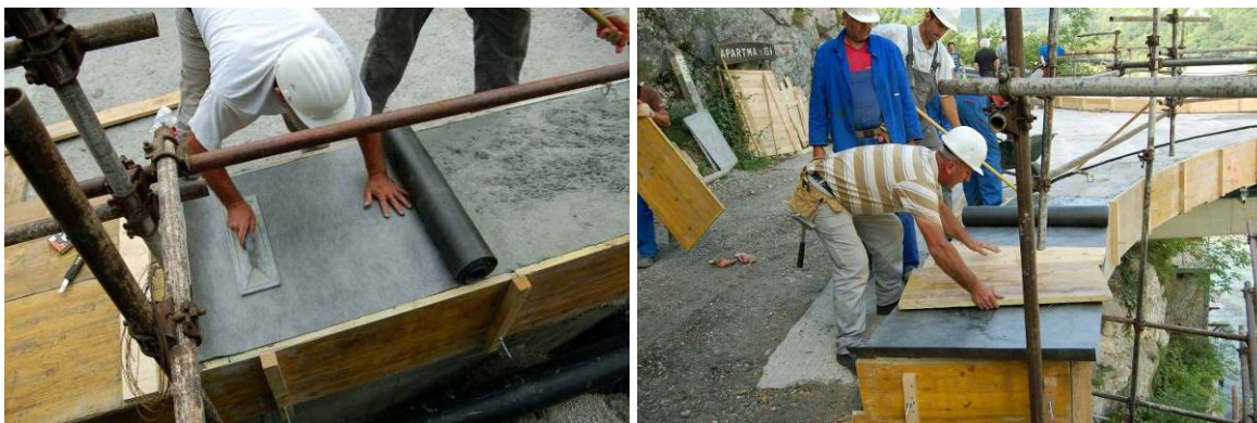
Figure 13: Surfacing of the UHPFRC for the footpath, over the ZEMDRAIN®.
