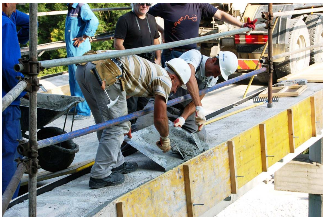
Figure 14: Pouring the UHPFRC CM32_11 for outer face of kerb.
