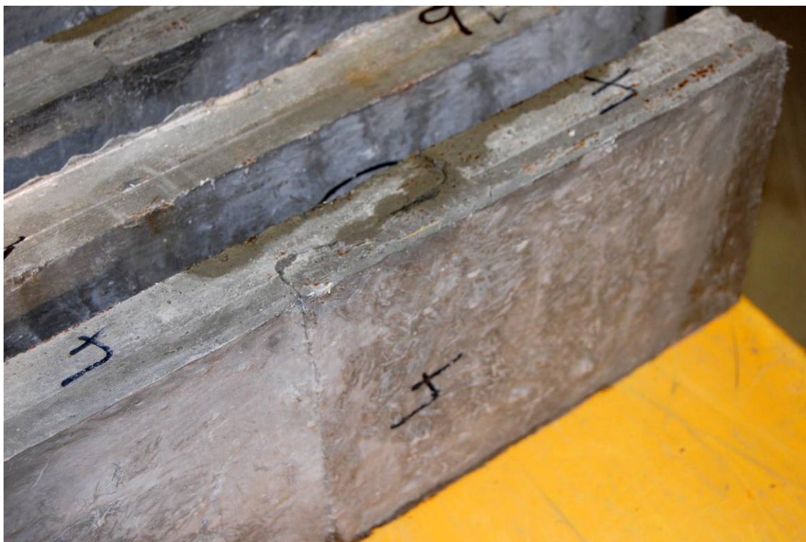
Figure 30: Leaking of water.
