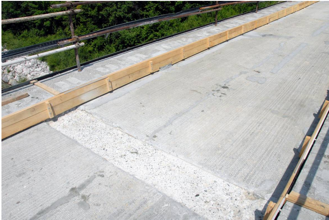
Figure 24: The transversal joint groove on the Log Čezsoški bridge.
