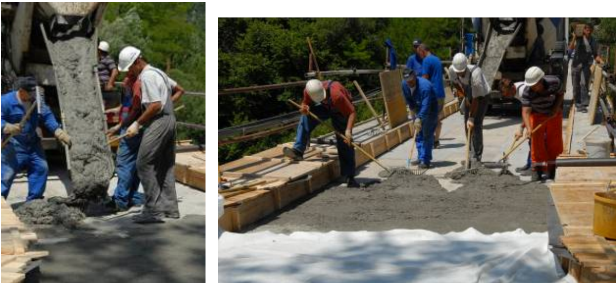
Figure 12: Application of the UHPFRC on the deck.
