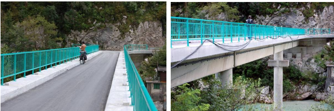
Figure 3: the bridge after the rehabilitation.
