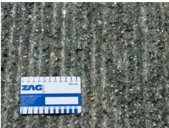
Figure 7: Surface preparation of the deck and footpath.
