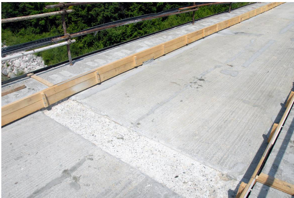
Figure 11: Groove for transversal joint at mid-deck surface.
