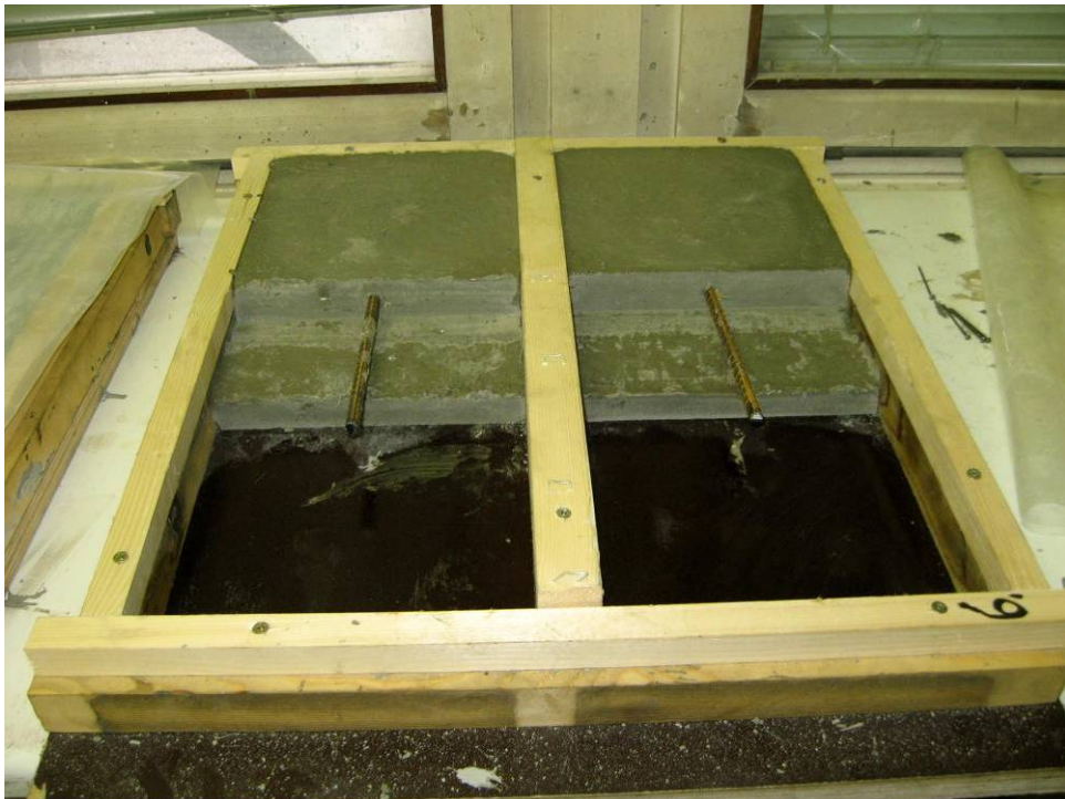
Figure 27: Position of the Re-bar in J06.
