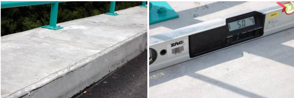
Figure 16: Detail of the footpath and slope of 5 %.
