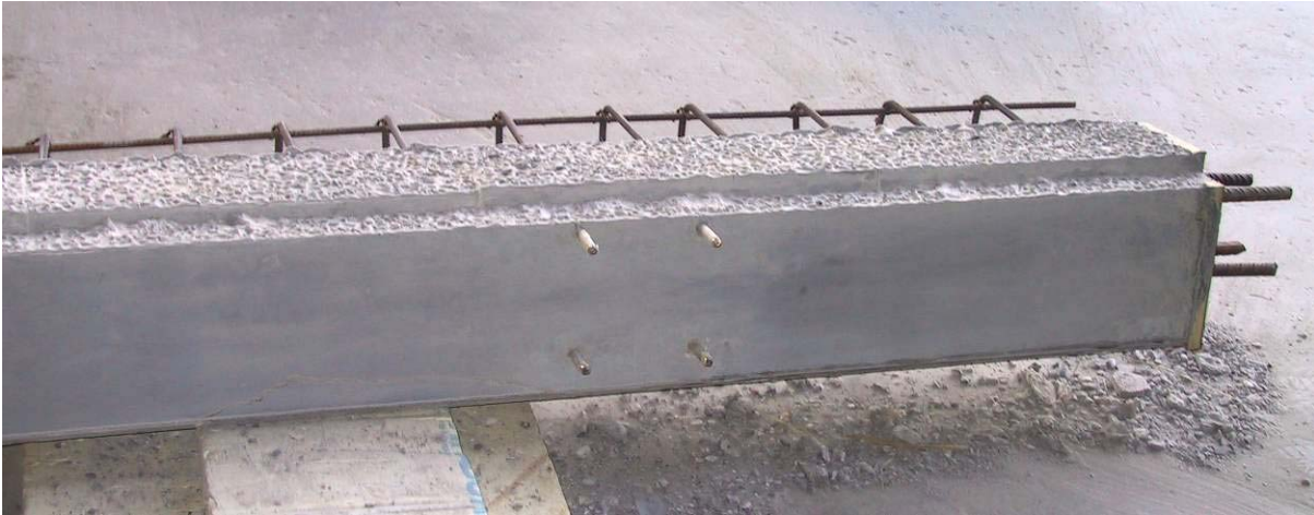
Figure 14: Prefabricated UHPFRC kerb segment.
