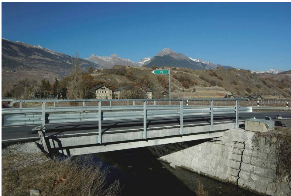
Figure 27: The Bridge in November 2004, after rehabilitation and widening.
