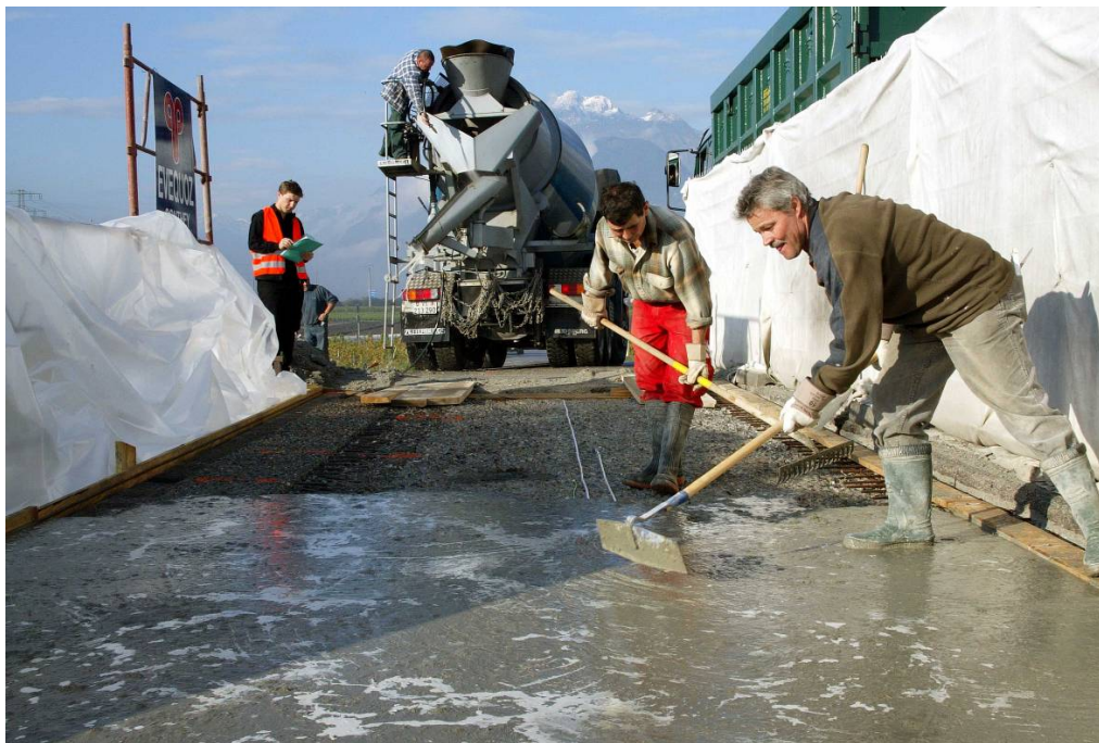
Figure 16: Overall view of the UHPFRC works (Photo A. Herzog).
