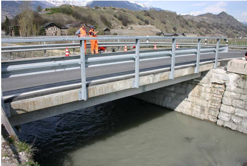
Figure 28: View of the bridge in April 2005, after rehabilitation.
