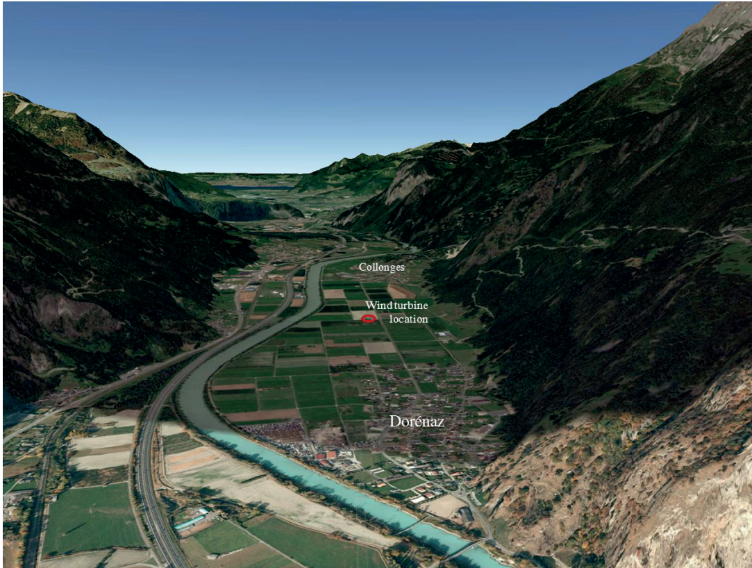
Figure 2.7 – Perspective view of the flat section of the Rhone valley in which the E-70 wind turbine is located ( 46^{\circ}09'35''\text{N } 7^{\circ}02'14''\text{E} ), as well as the villages of Collonges and Dorénaz. Map data: Google, DigitalGlobe.
