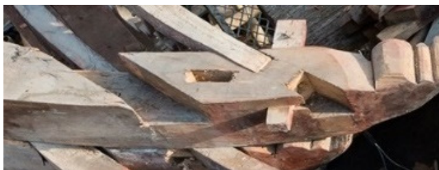
Figure 19. The wooden joinery of caisson in Ye's ancestral Temple, built in 1829, Ninghai, Ref. ZJ-07 © Xiaodong Chai
