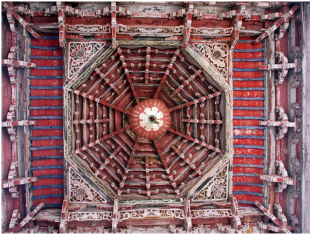
Figure 12. Octagonal type: opera stage of Chongxing Temple, Xidian Village, built in 1841. Height: 1.38 m; Diameter: 2.74 m. Ref. ZJ-05B © Peiliang Xu
