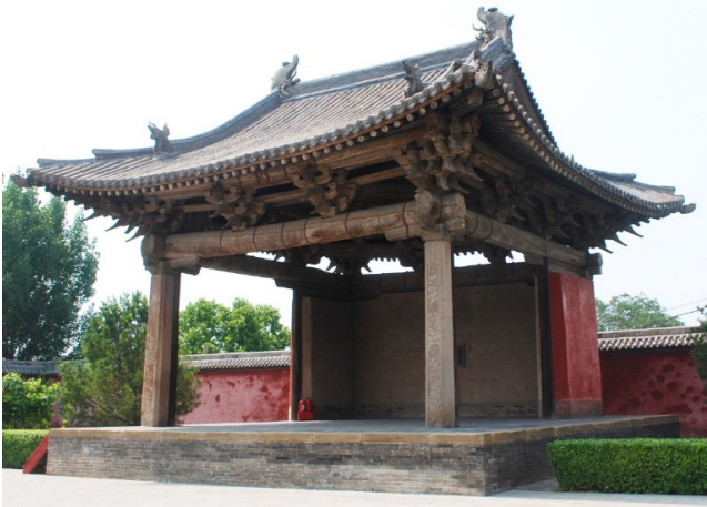
Figure 1. Opera stage of Niuwang Temple, built in 1283. Width: 7.45 m; Depth: 7.42 m; Height: 3.79 m. Ref. SX-01A © Jingxian Ye
