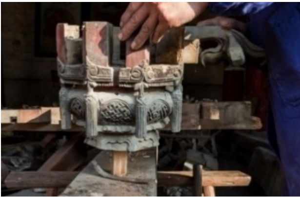
Figure 28. Manufacturing of new tenon tongue © Xiaodong Chai
