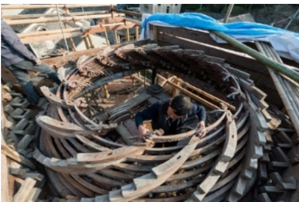
Figure 31. Close to completion © Xiaodong Chai
