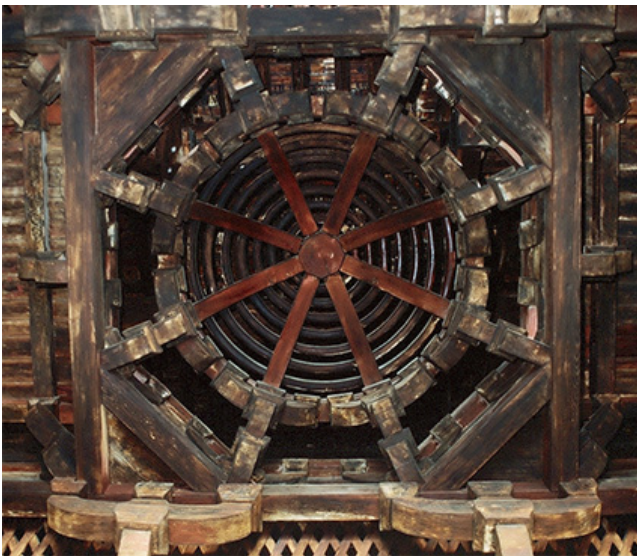
Figure 8. Douba type: the main hall of Baoguo Temple, built ca. 1013. Larger caisson: Height: 0.9 m; Diameter: 1.85 m. Smaller caisson: Height: 0.75 m; Diameter: 1.28 m. Ref. ZJ-01 © Peiliang Xu
