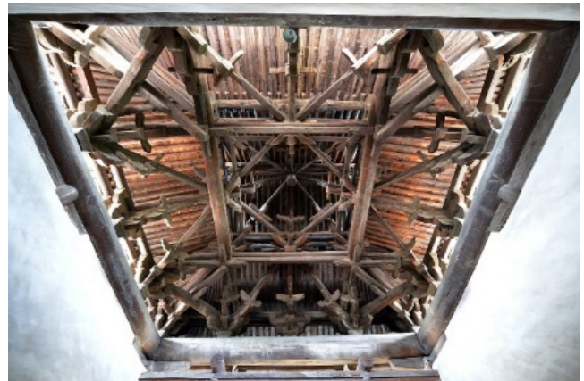
Figure 5. Caisson in Wangqu Temple, built in 1350 (est.). Width: 7.37 m. Depth: 6.83 m. Height: 4.14 m. Ref. SX-03 © Peiliang Xu
