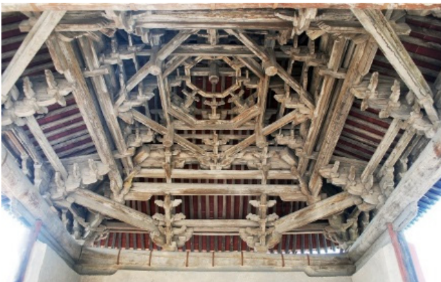
Figure 2. Caisson in Niuwang Temple, built in 1283. Width: 7.45 m. Depth: 7.42 m. Height: 3.79 m. Ref. SX-01A © Jingxian Ye
