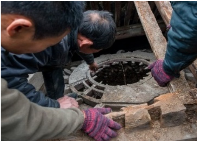
Figure 22. Removal of top plates © Xiaodong Chai
