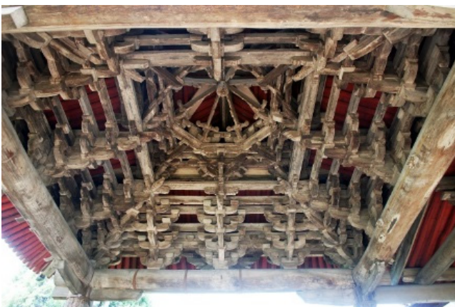
Figure 3. Second caisson in Niuwang Temple, built before 1283. Ref. SX-01B © Jingxian Ye
