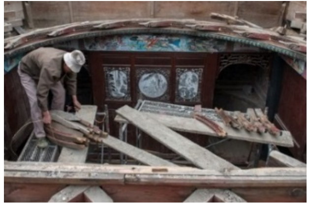
Figure 25. Same-layer components are tied up © Xiaodong Chai
