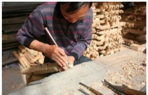
Figure 27. Carving of new cantilever component © Yi Zhou
