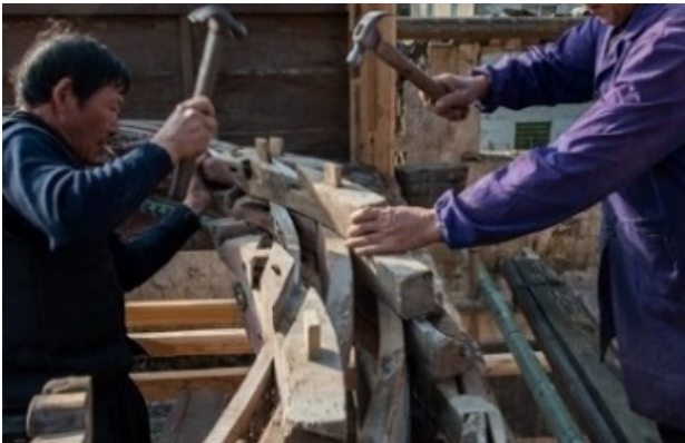
Figure 30. Hammering of the reassembled caisson © Xiaodong Chai
