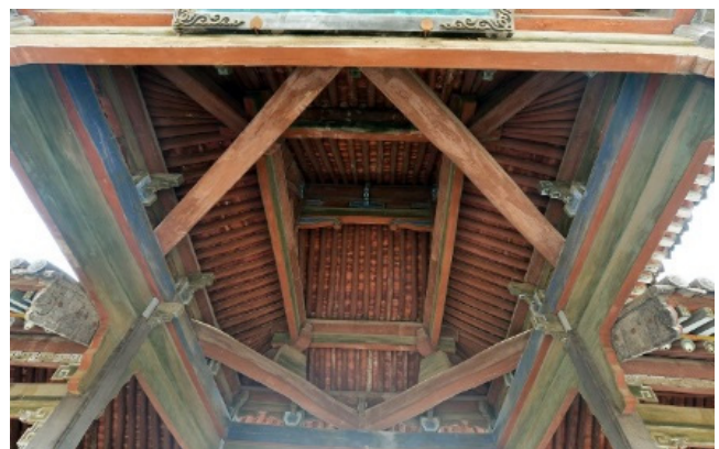
Figure 6. Caisson in the opera stage of Family Wang, built in 1700 (est.). Ref. SX-04 © Peiliang Xu
