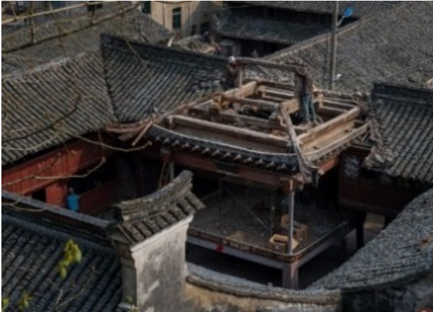
Figure 21. Disassembly of the roof © Xiaodong Chai
