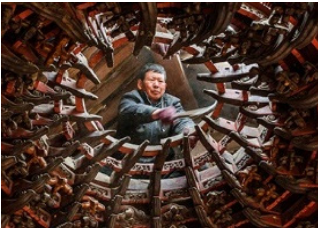
Figure 23. Hammering of the caisson © Xiaodong Chai
