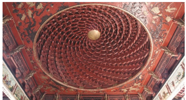
Figure 10. Spiral type: opera stage of Weishi Temple, Xiapu Village, built in 1890. Height: 1.15 m; Diameter: 3.3 m. Ref. ZJ-03 © Jingxian Ye
