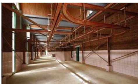
Ouahigouya, inside the municipal slaughterhouse (photo SDC)
