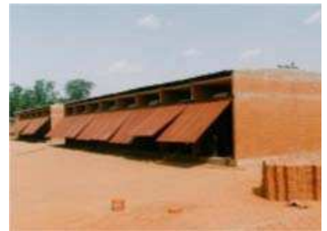
The market of Ouahigouya, un building in local materials (BUCO-DDC Ouagadougou)
