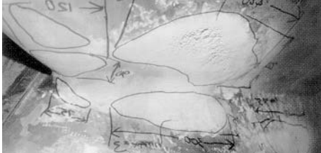
Fig. 26 Typical erosion at the wall of the blade suction side due to inlet edge cavitation, shaded area A of Fig. 25.
