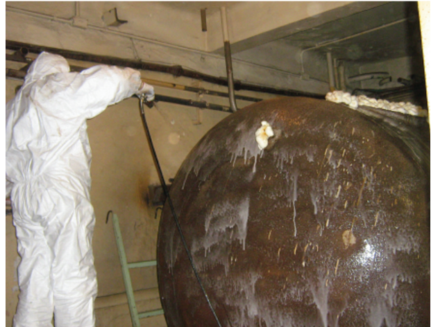
Figure 5. Applying polymer localizing coating.
