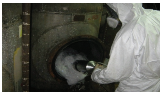
Figure 8. Foam decontamination of the internal equipment surfaces.
