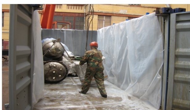
Figure 7. Loading of the large-sized radiation-contaminated equipment into the PU-2ETS-ST transport containers.
