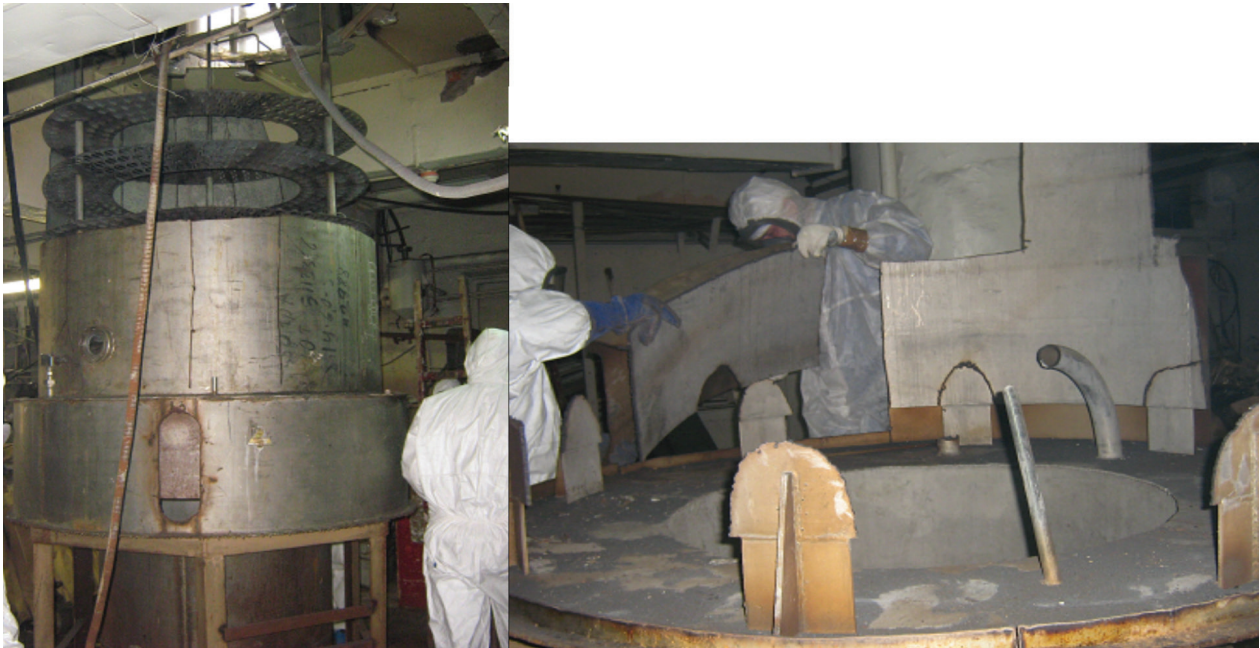
Figure 3. Removal of the column-type equipment.
