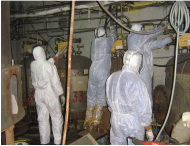
Figure 2. Dismantling the process pipelines.
