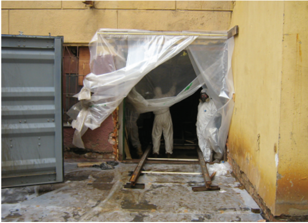
Figure 4. Opening in the wall of the radiochemical facility; crane runways.
