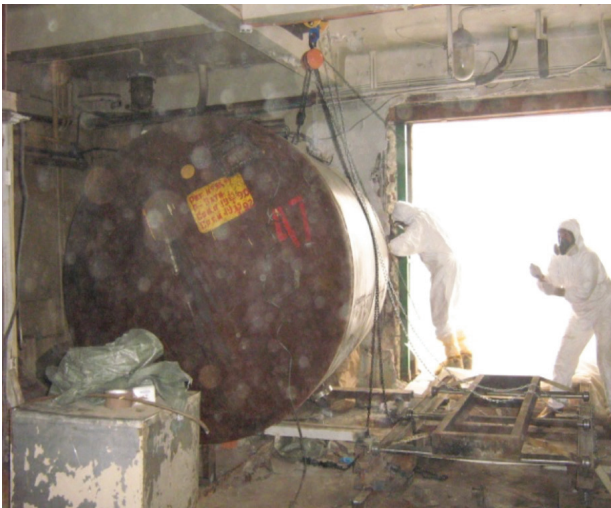
Figure 6. Dismantling and removal of the large-sized capacitive equipment.
