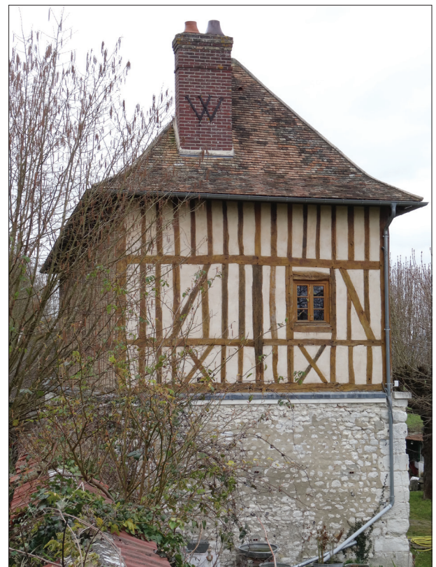
Plate 8 — House at Vernonnet, Normandy. The coyeau form of the roof probably reflects replacement of thatch with tiles.
