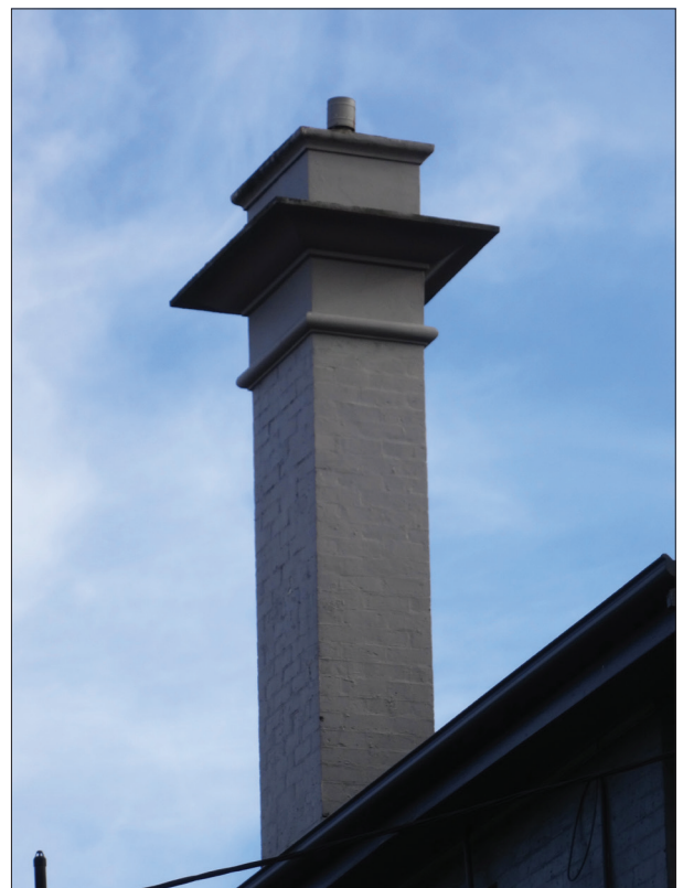
PLATE 5. — A. Harold Masters: chimney-stack, Newstead Hotel, Launceston.
