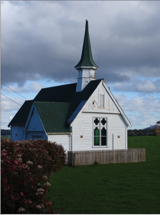
Plate 12 — St Alban, Pipers River, a characteristic wooden country church by Alexander North; in this case the spire surmounts a false belfry.
