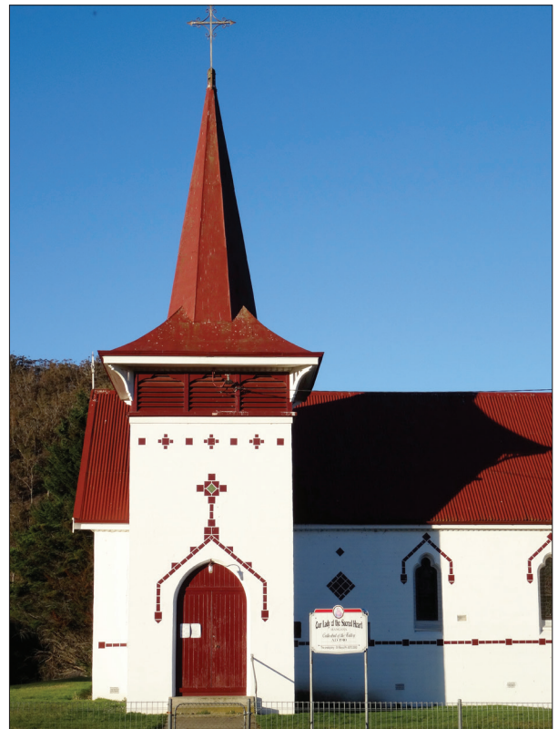
Plate 11 — Our Lady of the Sacred Heart, Mangana, a concrete church for a gold-mining town, decorated with inset glazed tiles.
