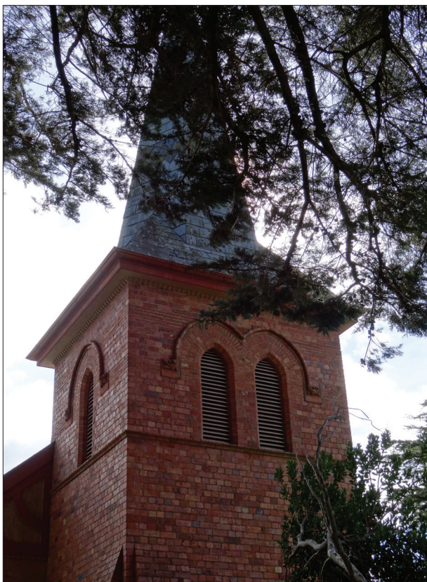
Plate 9 — St Peter's, Nile, brick tower and slate-covered spire.
