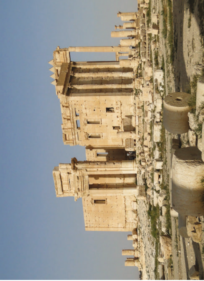
Figure 7.8 The Temple of Bel in Palmyra (Syria), first century CE. The temple shows a typical Greek-Roman peristyle around the central building, which, in contrast to the Greek-Roman tradition, presents an entrance on the long side as well as decorative merlons on the top, both features recalling Near Eastern traditions (Gagnon 2010)
