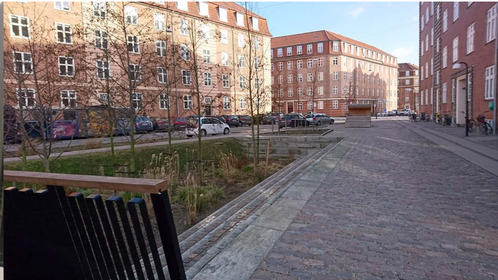
FIGURE III. DETENTION STORAGE IN TÅSINGE PLADS, COPENHAGEN.
