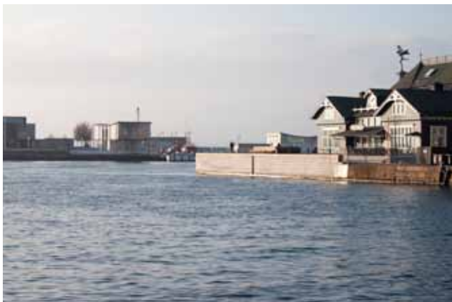
Figure 70 - The recently developed area around the 'New Tivoli' has been raised in expectance of sea level rise. The great height difference makes the relationship to the water more distant.
