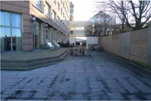
Figure 84 - The walk connecting the future bridge to the dock today.
