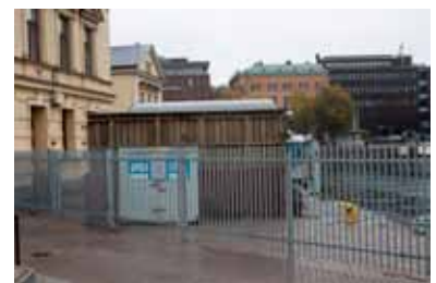
Figure 24 - Trying to reach the water is unrewarding. Finding a fence around Tullhuset serving as a barrier demanded for its role in international transportation.
