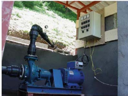
Figure 3-3 A centrifugal PAT-based pico hydropower station, installed in the West of Iran [4]
