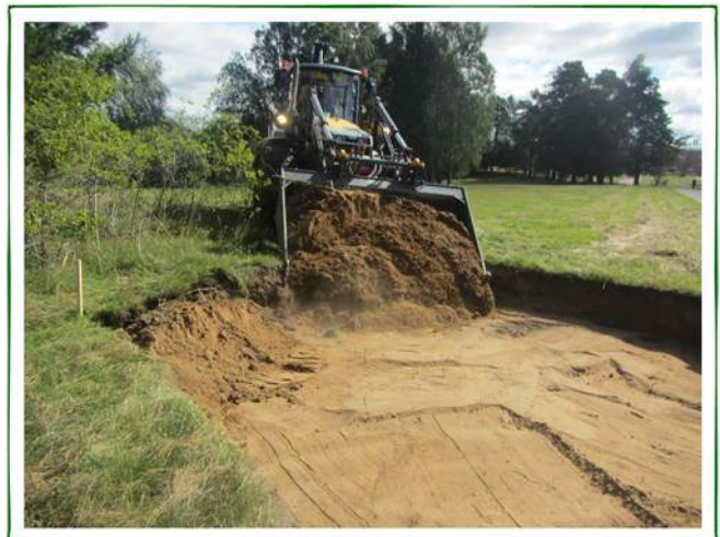
Moving sand with a backhoe © Niina Sallmén
