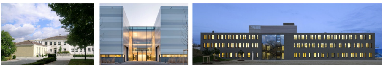
Figure 1.1-1 Microwaves and Radar Institute: main building (left) and TechLab (middle and right)
