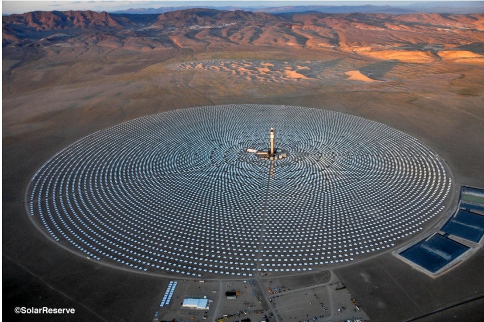
2 Figure 2: 110-MWe Crescent Dunes tower CSP plant in Tonopah, Nevada, USA, with 10 hours of 3 thermal storage in ~32 000 tons Solar Salt. (source: SolarReserve)
