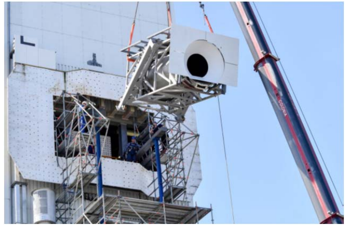
FIGURE 2: 2.5 MW TH PROTOTYPE DURING INSTALLATION IN THE JUELICH SOLAR TOWER
