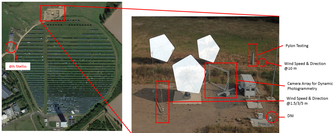
FIGURE 2. Juelich Solar Field with heliostat testing platform (Helitep, left). Equipped with one Stello (in the front), two additional ones with designated foundations (in the back) and a 4th heliostat in Western location for different main angle setup.
