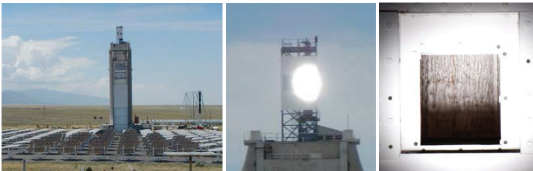
FIGURE 1. Images of 1 MW t particle-receiver system tested at Sandia National Laboratories.
