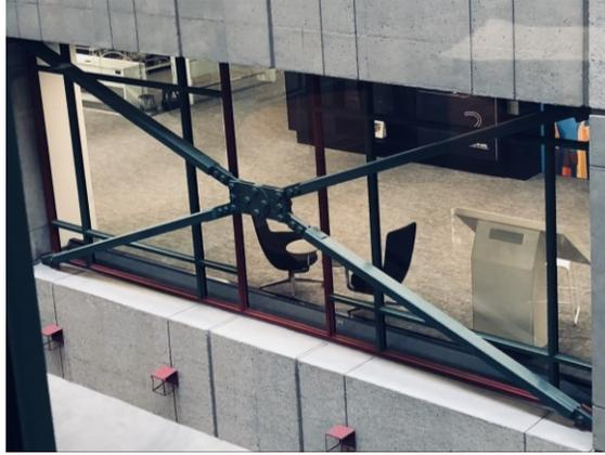
Figure 1-2 Pall Friction dampers installed in the Webster Library of Concordia University, Montreal, Canada.
