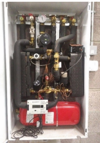
Figure 4-18: The Dual Heat Exchanger Sub-System
