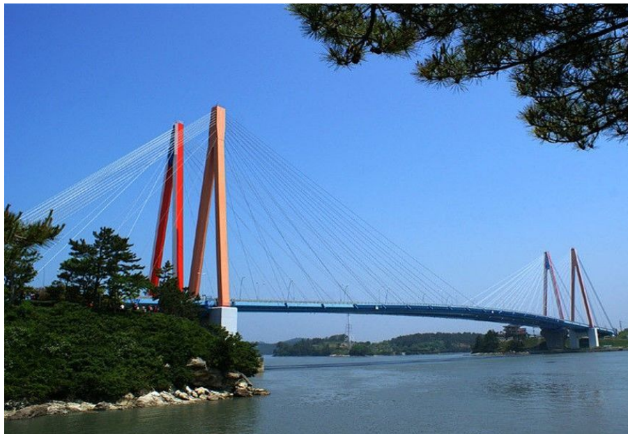
Figure 2-7: Jindo suspended bridge which is equipped with a TMD by TESolution company - South Korea (TESolution www.tesolution.com , June 2018)
