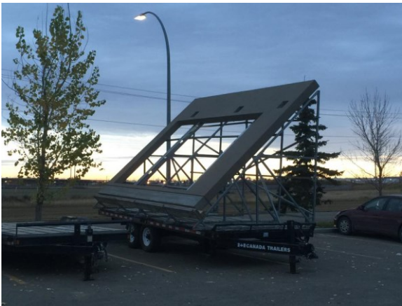
Figure 4.19: Alignment of panels on trailer
