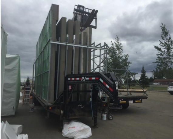
Figure 4.19: Alignment of panels on trailer
