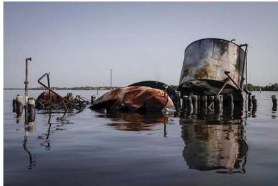
A broken oil platform in the lake. PHOTO: FABIOLA FERRERO FOR THE WALL STREET JOURNAL
