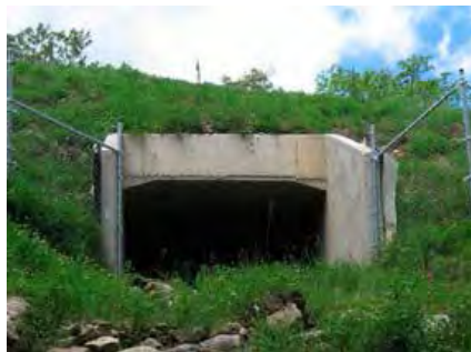
Figure 8.4. Correct installation of the fence makes the entrance easier to locate by fauna. Photo: M. Fernández Bou.
