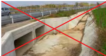
Figure 9.9. Canal fences prevent animals from returning to the surroundings. Photo: F. Navàs.
