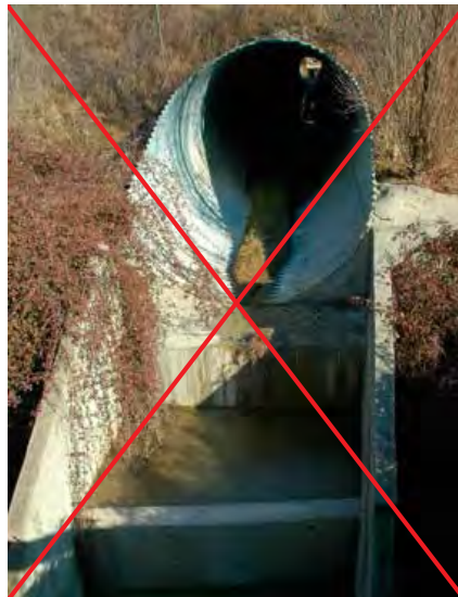
Figure 9.11. Stepped outlet: a trap for wildlife. Photo: F. Navàs.
