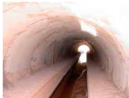
Figure 9.4. Interior of a culvert with dry lateral ledges. Photo: F. Navàs.
