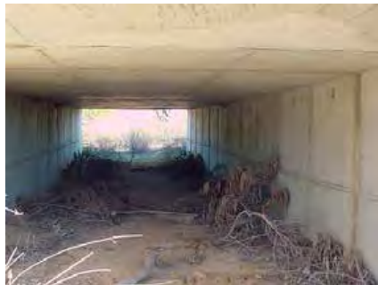
Figure 8.2. Rows of dry branches provide shelter for small animals. Photo: P. Robles.
