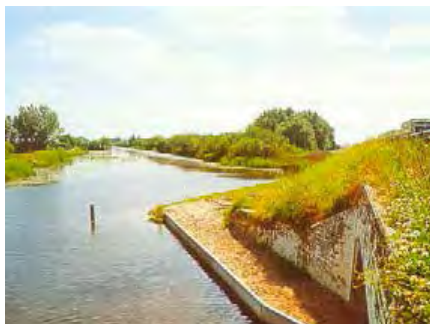
Figure 9.3. A ramp facilitates optimal connection between the dry ledges in the culvert and the surrounding natural habitats. Photo: H. Bekker.
