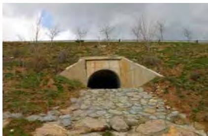
Figure 9.7. Stone bed replacing a stepped culvert outlet. Photo: C. Rosell.
