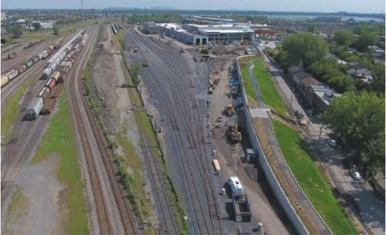
Fig. 14. Aerial view of rue de Sébastopol showing sound berm with central ramp and lookout. Date unknown. Private collection of Carl Dettman.
