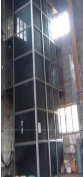
USTC stairwell shaft
