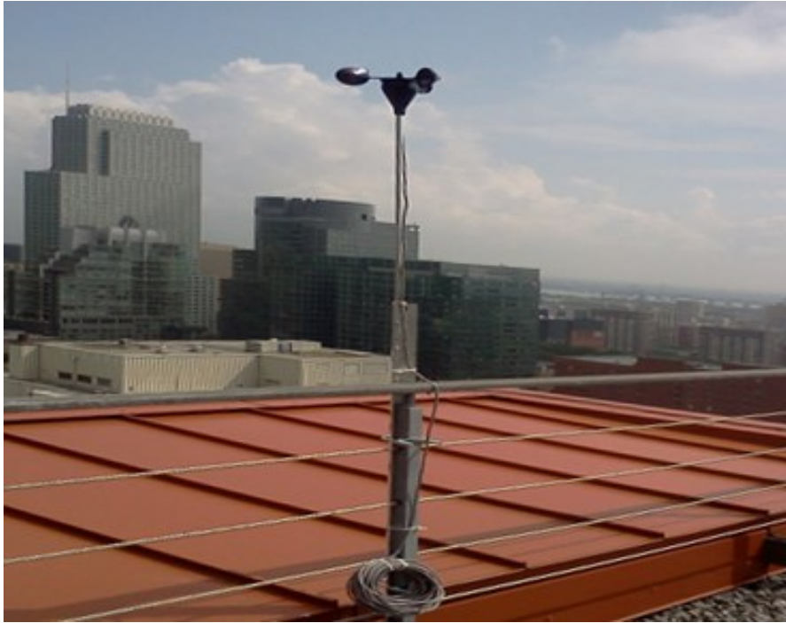
Fig. 2. 12: Installed Anemometer above the Roof of the EV Building.
