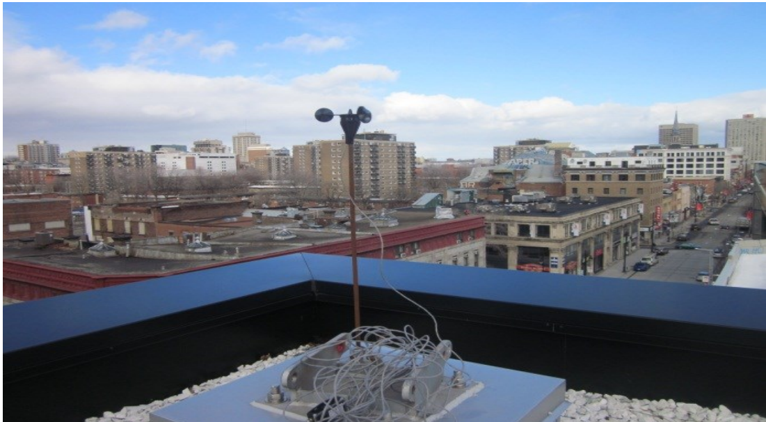
Fig. 2. 23: Installed Anemometer over the Roof of Equiterre Building where the North is toward the Corner of the Building.
