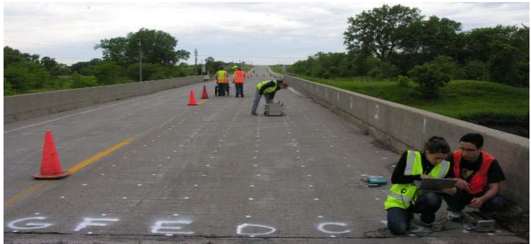
Figure 4-3. 2 ft. x 2 ft. grid (Gucunski et al. 2011)
