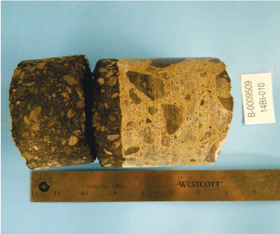
Figure 5-27 Corroded coring sample
