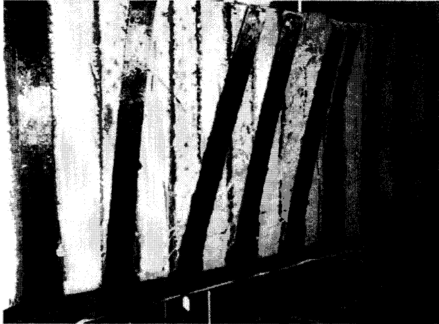
Figure 2.9 Debonding failure of beam strengthened by U-jacket CFRP strips (Leung et al., 2007)
