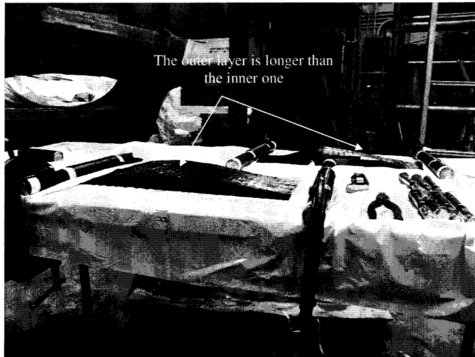
Figure 5.14 Anchor of beam B-2 while being manufactured
