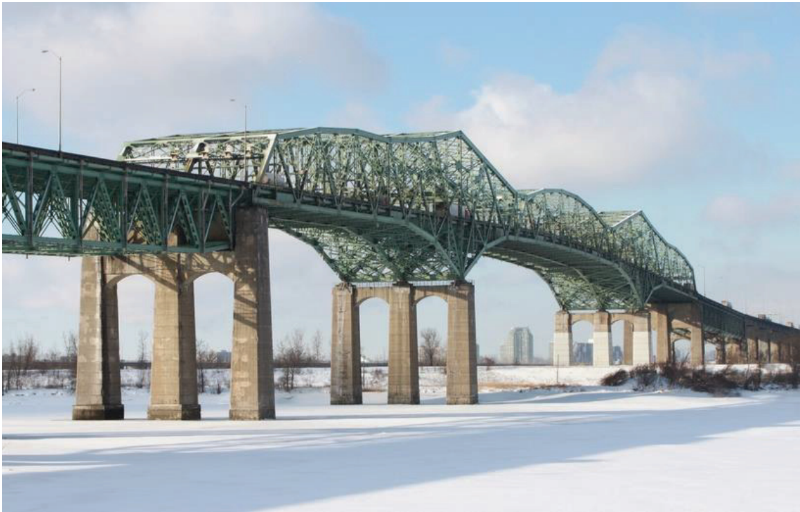
Figure 49: Side View of the Champlain Bridge
