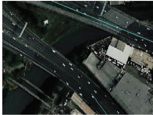
Figure 46: Overwater Bridge Areal View
