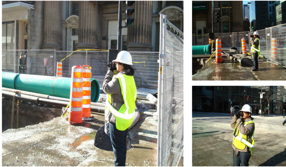
Figure 4-1: Image collection from construction sites
