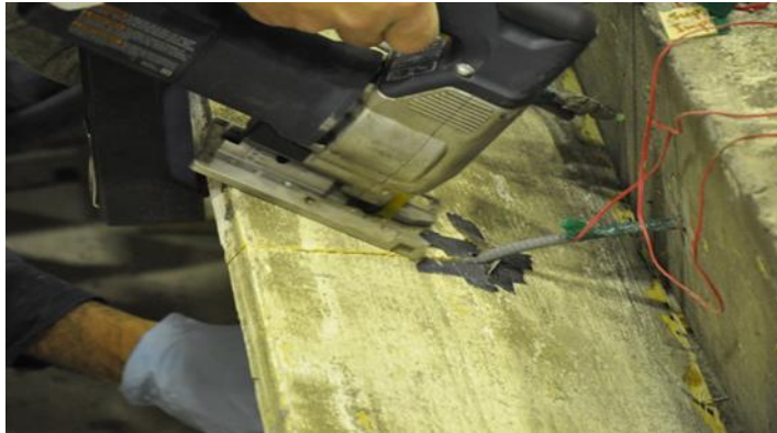
Figure 3-6 Stripping form-work
