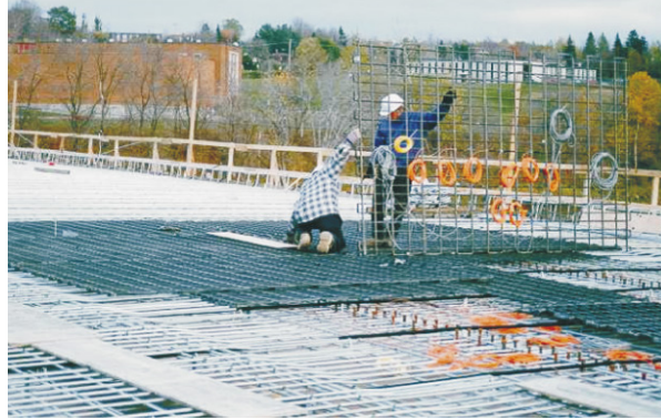
Figure 2-2 Instrumented CFRP grid during the installation (Benmokrane et al., 2000)
