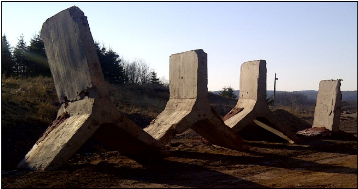
Figure 2.8. Folded-Plate Shell Footings. Potash Corp., Sussex, NB, Canada.
