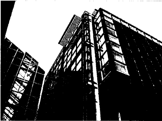
Figure 2-7: Red River college's integrated STPV façade (Boake 2007)
