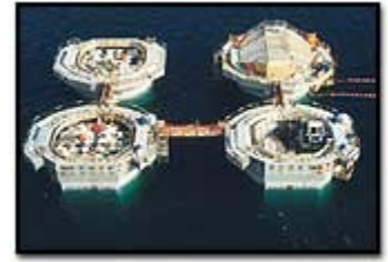
Gravity Base Structure
