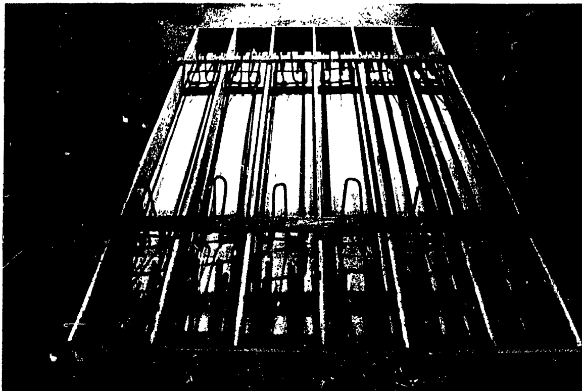
Figure 4-3 View of the wood form
