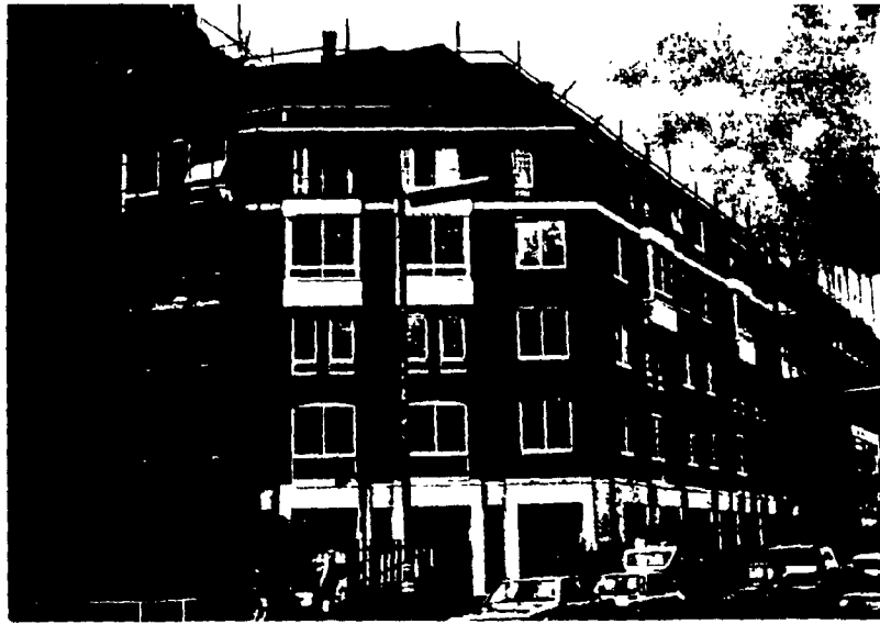
Fig. 2.10 At Ebury Street, London (1977). 96 Luxury Flats structure (24,000 tons) supported on 1400 elastomeric bearings (Courtesy of Liquorish A.D., Director Tico Manufacturing Ltd.)
