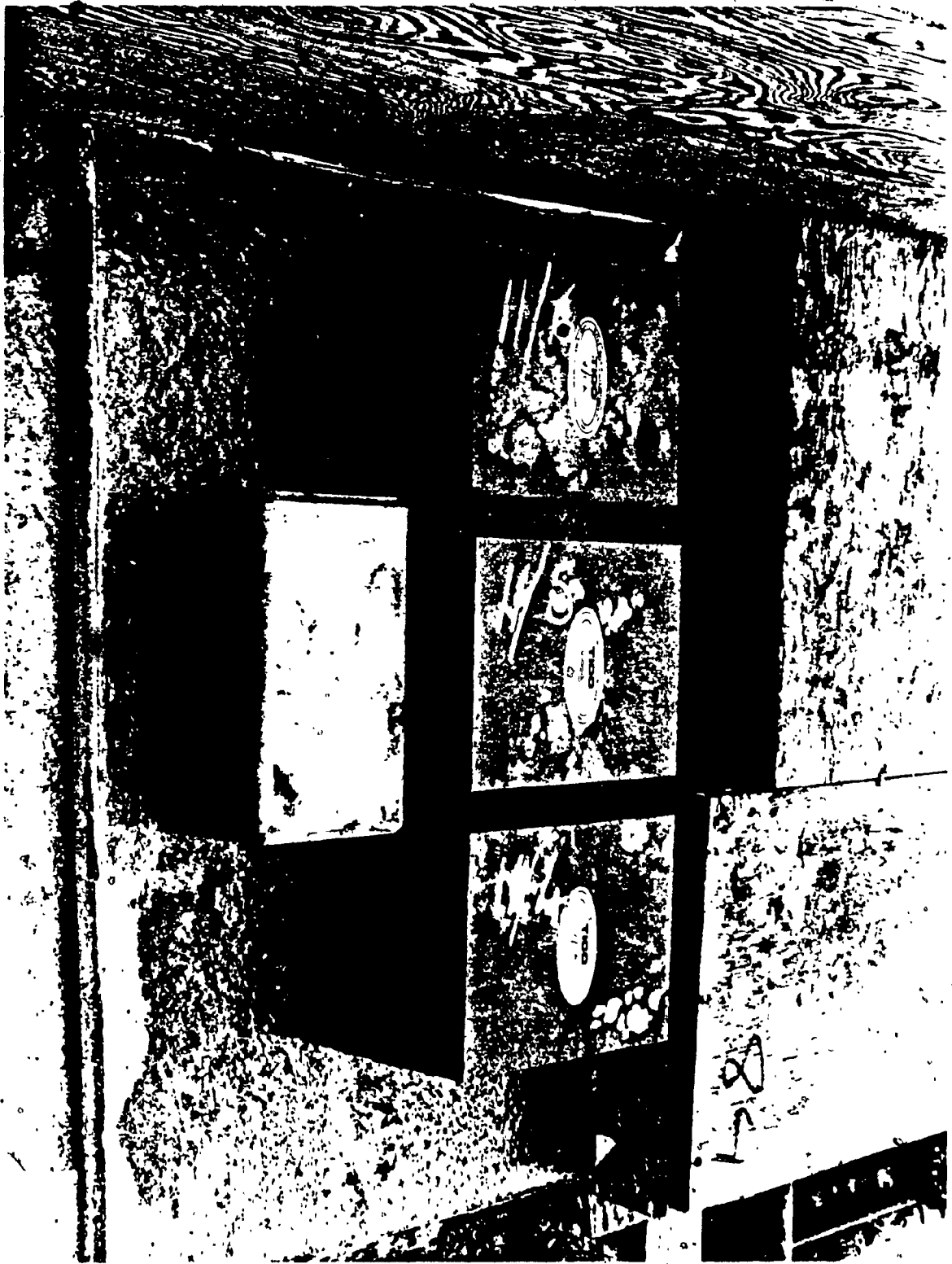
Fig. 1.3. A typical steel laminated Bearing Pad unit, in position.
