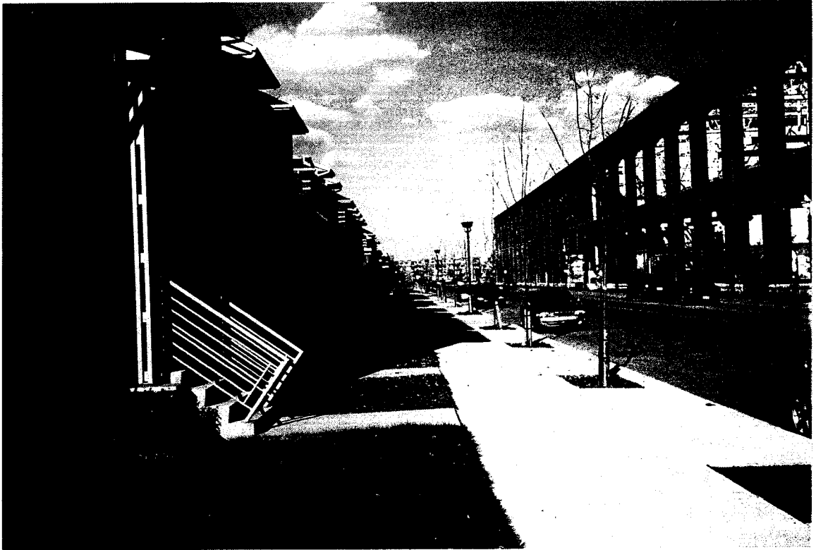
Figure 5. Façade of former Angus Locomotive Shop. Photo taken by author October 2002.
