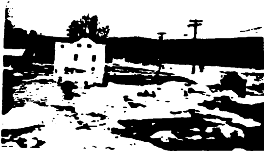
a) Flooding of towns
