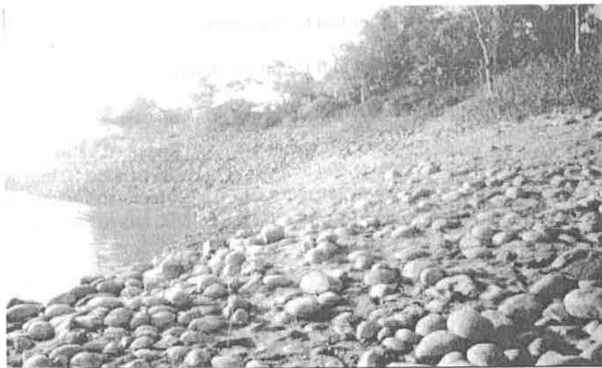
Figure-5: Bank Protection Embankment, location Kanishail to Ghashitula
