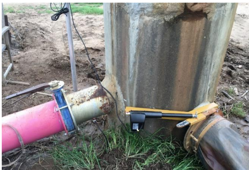
Figure 6-19 – Main supply line from pump and initial PST installation (Feb 2016 - Sept 2016) at Linton Site.
