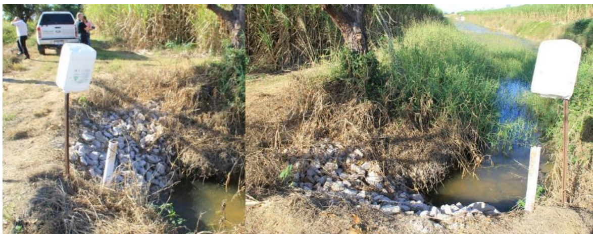
Figure 6-13 – Drain at corner of block 1 at Pozzebon site.
