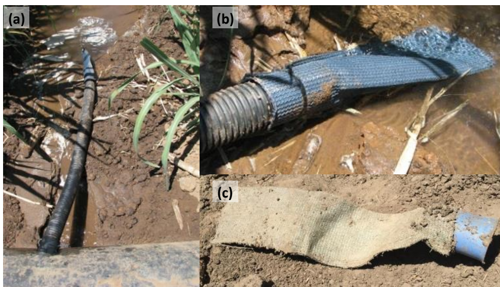
Figure 5-3 – Examples of sock outlets (a & b) corrugated drainage pipe sock (c) cup and fabric sock
