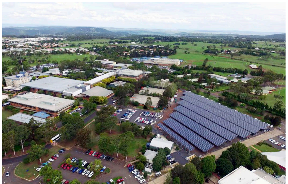
↑ Making good use of a car park space: the largest solar car park in Australia—3842 panels and over 1MW!—is now operating at USQ's Toowoomba campus, providing energy and shading.
