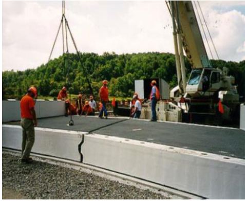
FRP Slab Bridge over Bennetts Creek New York, USA (Stewart 2011)
