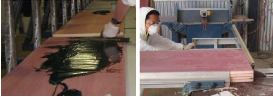
(a) Gluing of sandwich panels
