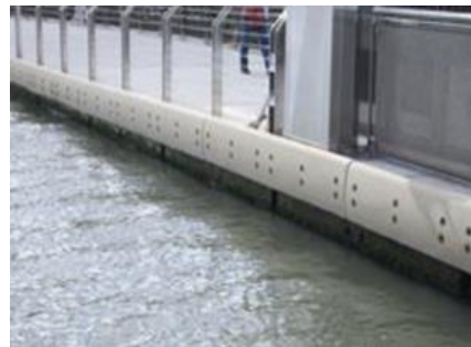
Fibre composite Waler, Australia (Aravinthan 2012)
