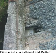
**Figure 2.6 -** Weathered and Rotted Timber deck Planks
