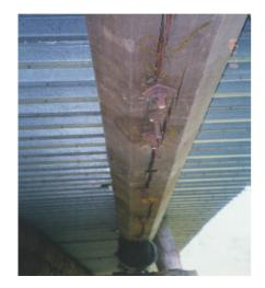
Figure 2.4 - Splitting in Girder
