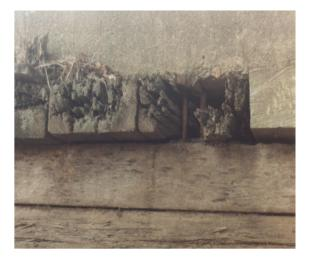
Figure 2.5 - Rotted Ends of Deck Planks
