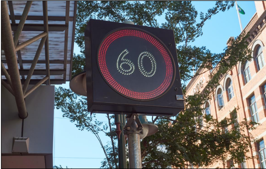
Figure 2.7 – Variable Speed Limit Signage in Fortitude Valley
