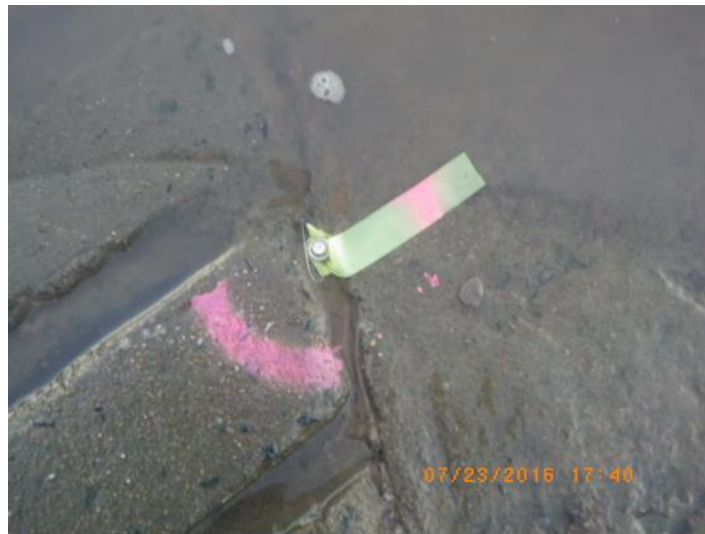
Datum pin set at nominated navigable level
